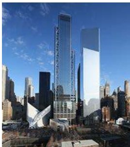
24_ Rogers Stirk Harbour + Partners_3 World Trade Center_New York_Silverstein Properties Inc. - Joe Woolhead
